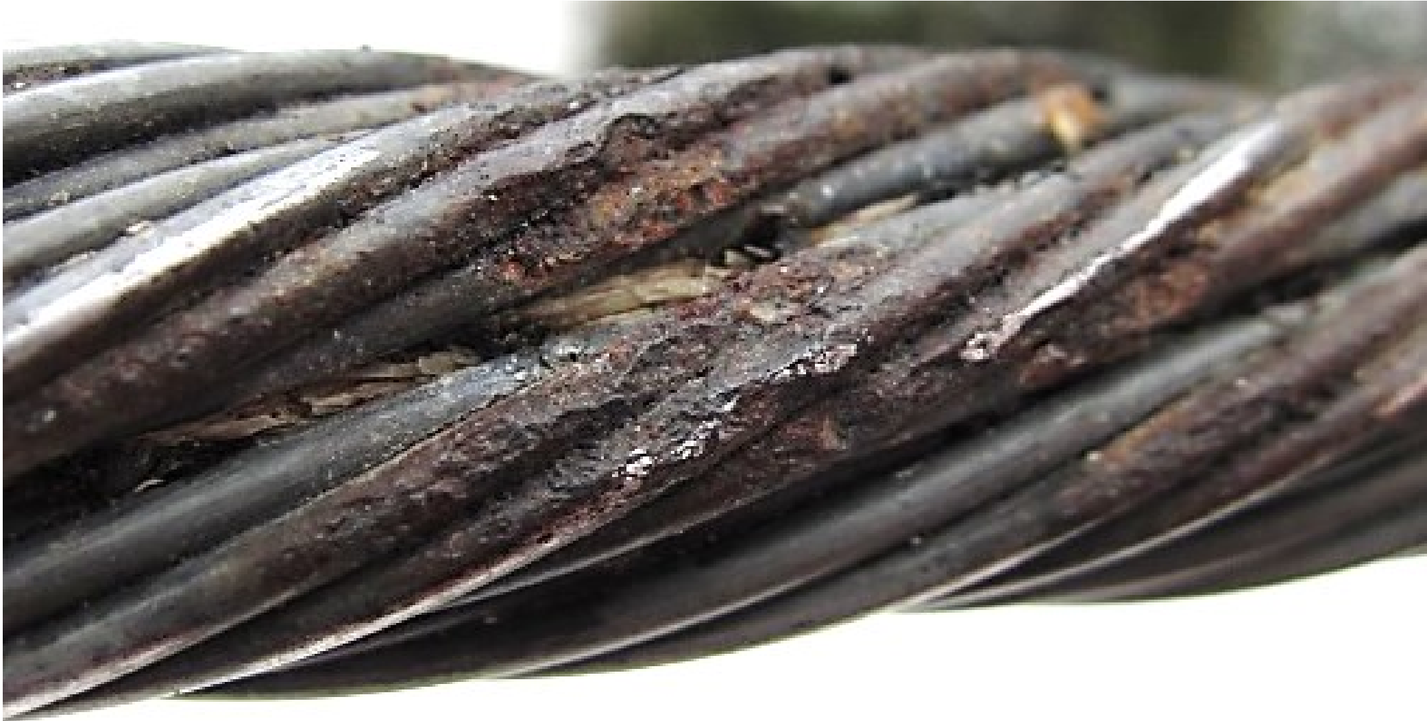
Wire breaks due to corrosion
