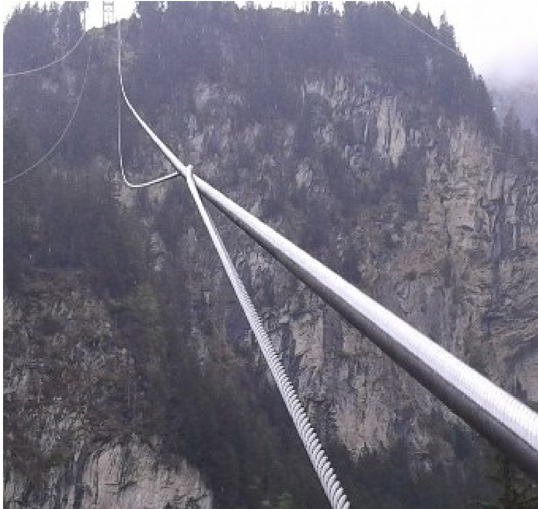
Rollover of a hauling rope
